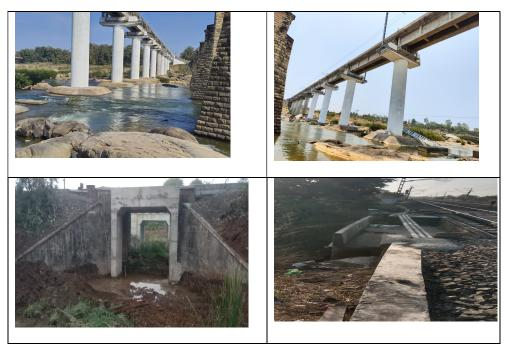
2 The work of strengthening to abutment & wing wall of Bridge no. 29 DN between KNHN – KP on A route has been done by pressure grouting and Pointing.
