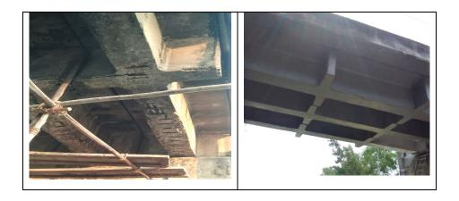
The work of re-building of small opening bridges Nos. 9A & 9C in TMR – TRDI section have been done by construction of RCC box in place old arrangement.
