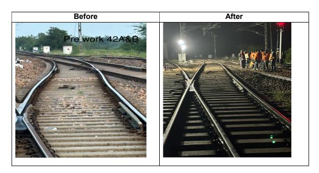
The work of 2 No. crossover layout corrections have been done with T-28 machine at Itwari & Rewral yards. In crossover connecting point Nos. 65A & 65B and 153 A & 153B respectively has been done.
