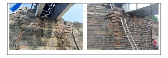
At bridge no. 31 DN ( ORN-3 bridge ) between KNHN – KP, tilted ballast retaining wall dismantled and gap between 3rd line bridge & DN line bridge is covered with RCC slab with clear joint.
