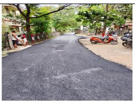
Construction of approach road at Pipardahi railway station in NIR – CWA section to the extant of 370 mtr X 4 mtr has been done.
