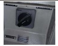
*Fig. 18(13)* HBL: Kavach Isolation switch at BIU unit
