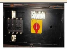
Fig. 17(15) Medha: Two nos. Of MCBs at onboard Kavach
