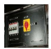
Fig. 17(18) Medha: Two Nos. of MCB at Onboard Kavach
