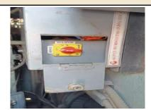
Fig. 18(12) Kernex: Kavach Isolation switch
