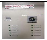
*Fig. 18(3)* HBL: Isolation switch on BIU box
