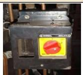
Fig. 18(9) Kernex: Kavach Isolation switch atPn.panel
