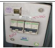
Fig. 17(17) HBL: Kavach MCB(two) besides Pneumatic panel
