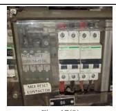
Fig. 17(9) HBL: Two nos. Of MCBs at SB-1 PANEL
