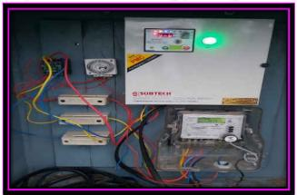
3) 02 Nos. 10KVAR capacitors have been provided at Sewage treatment plant/ITR for improvement of power factor.
