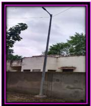
5) 43 Nos. new SST electric poles having 45W LED light fittings have been provided with 600 mtrs. 4x16 sqmm cabling work WS/MIB.
