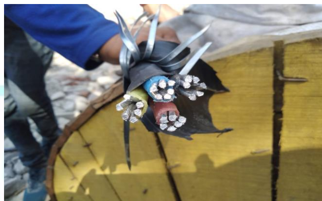
Middle of cable 6 strands
