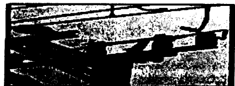
ISOLATOR IN CLOSED CONDITION (SUPPLY ON)
