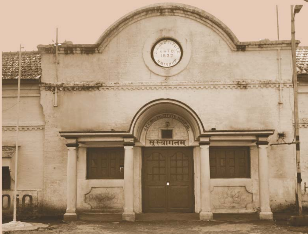
Railway Institute Nainpur : This building was constructed in the year: 1922. All Indoor game facilities were provided. Even now the building is in a sound condition.
