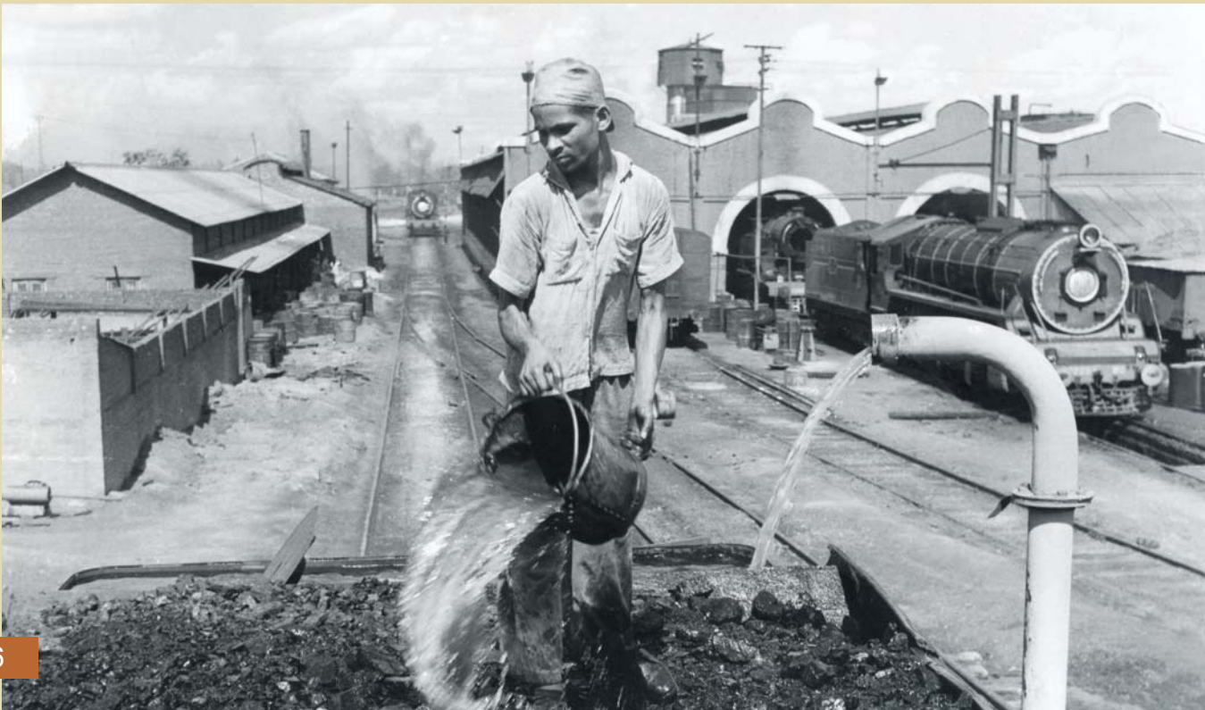
Second Firemen wetting the coal for increasing the fuel efficiency
