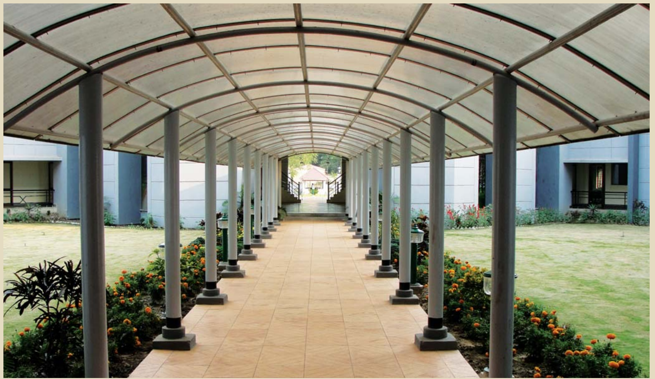
Aisle between Block 'A' & 'C'
