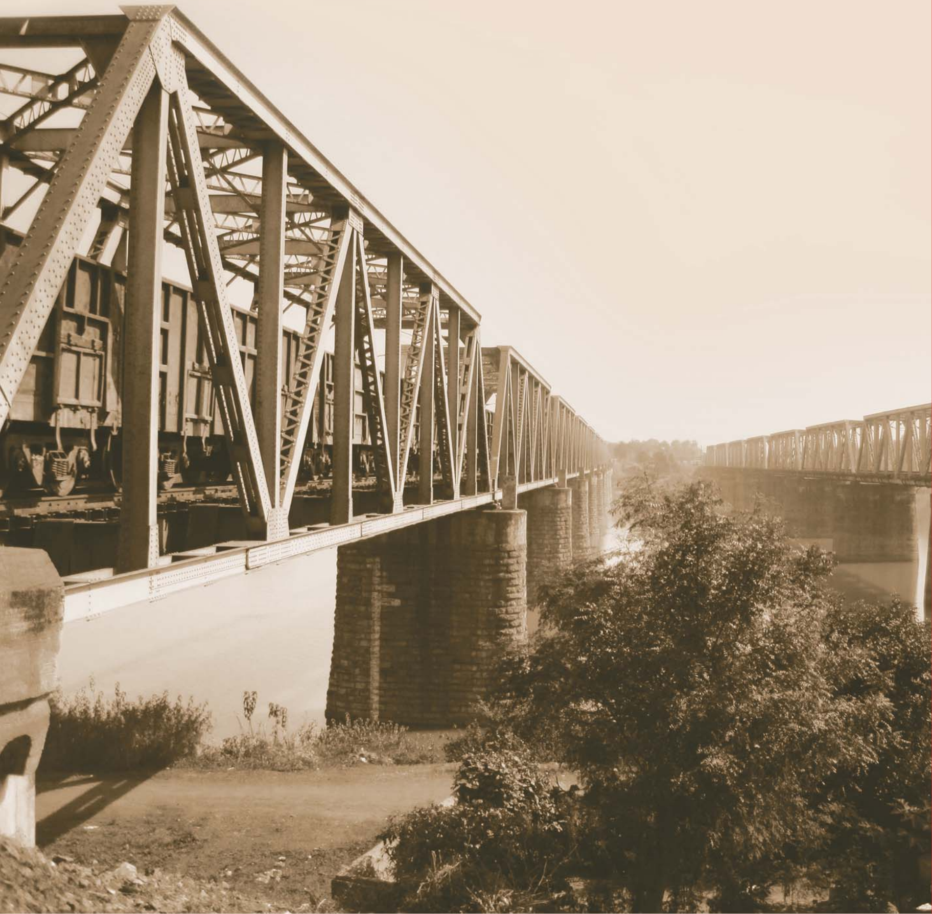
Bridge No.182 on IB river, constructed in the year 1887. It has 2 X 40 plate girder and 9 X 150 feet open web girder of total length 435m well foundation. The Mahanadi reservoir is located downstream of this bridge.
