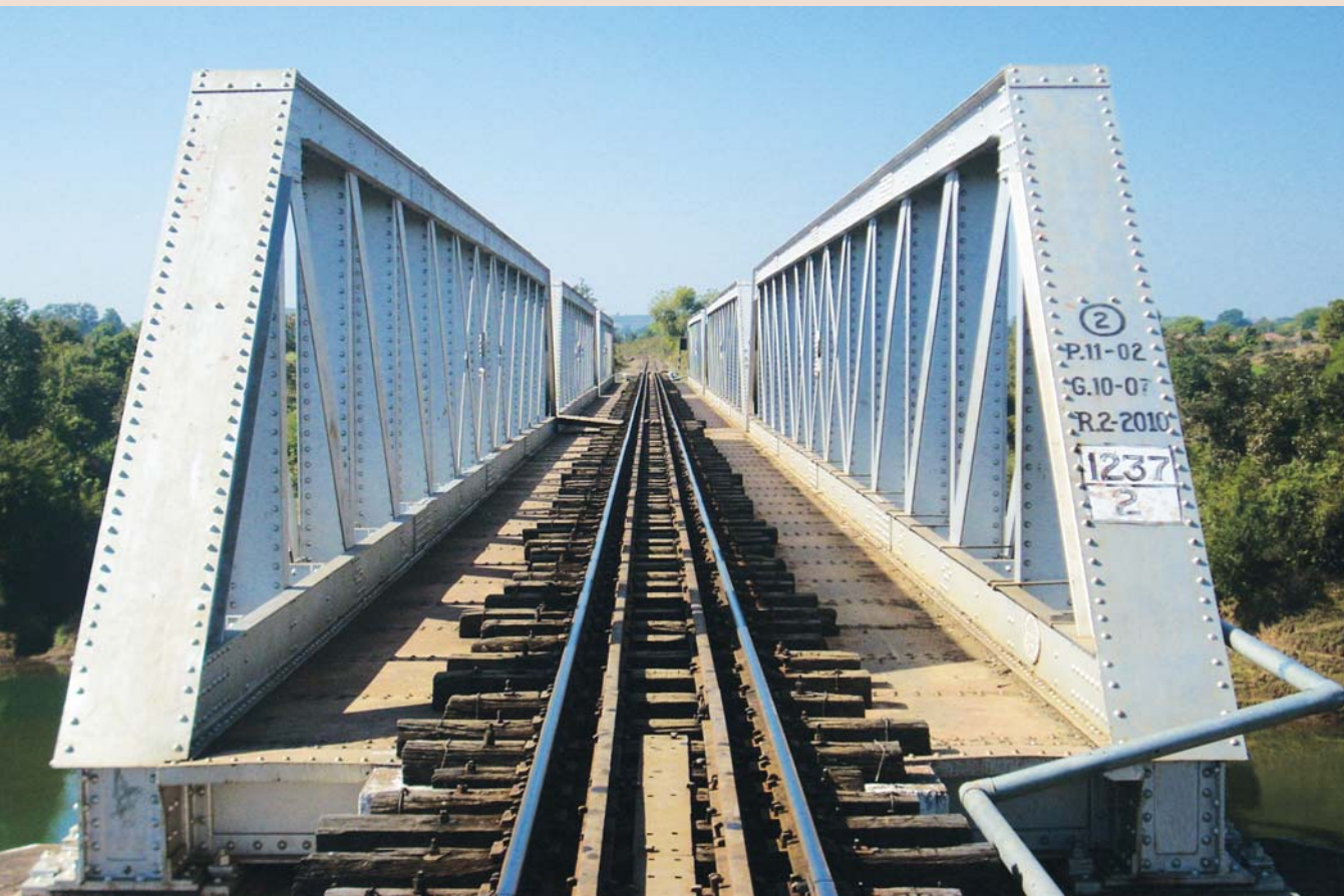
Bridge No. 153 near Karaboh Station on Pench River, was constructed during 1902- 4 (Girders' built year: 1903). Highest Flood Level ever recorded on Aug 1, 1913 was 1'6" above rail level.
