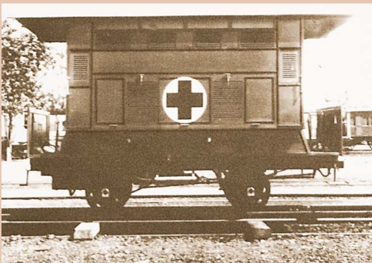
Self propelled (Petrol Engine Driven) Ambulance Car built in 1930
