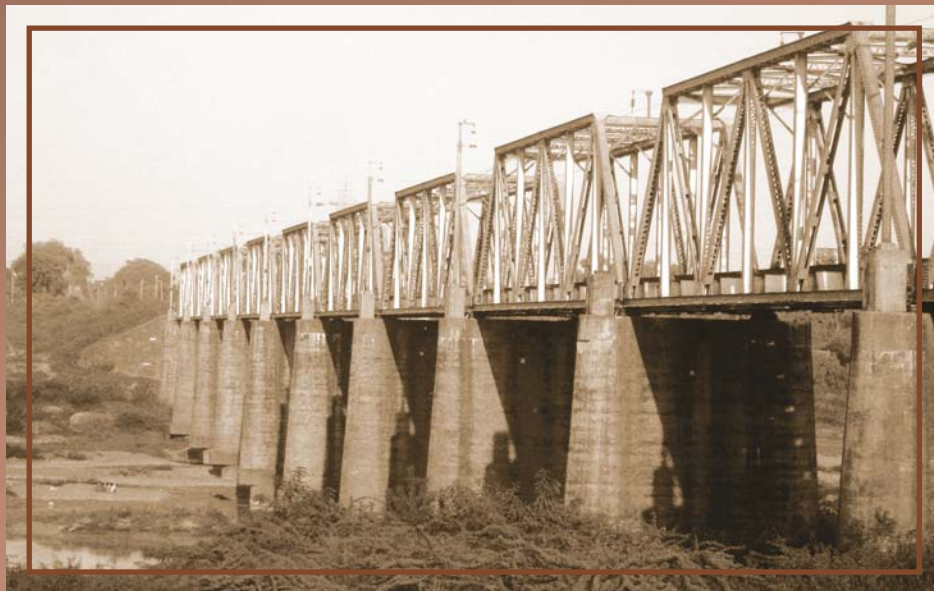
Hasdeo River Bridge No. 63 constructed in the year 1963 while connecting Gevra with a rail link. It has 2 X 40 feet plate girders + 10 X 100 feet open web girders.
