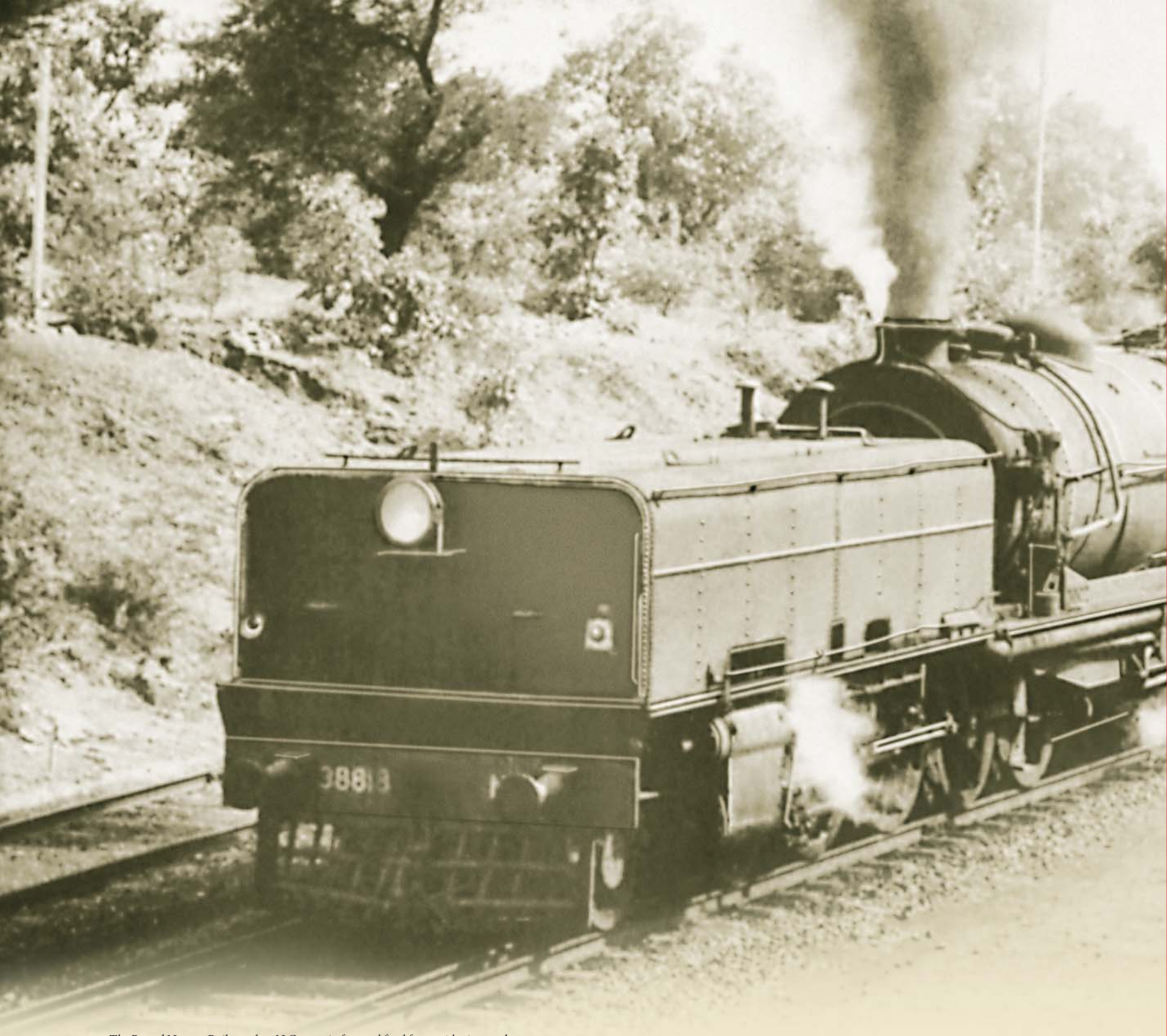
The Bengal Nagpur Railway class N Garratt in first and final form, with piston valves. Indian Railways No. 38818 leaves Kusumkasa loop in 1970, with a 2400 tonne ore train bound for Bhilai steelworks.
