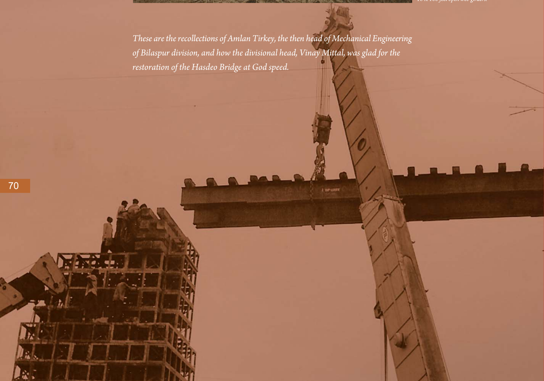
Hasdeo River Bridge No. 63 constructed in the year 1963 while connecting Gevra with a rail link. It has 2 X 40 feet plate girders + 10 X 100 feet open web girders.
