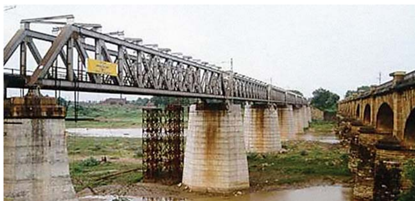
Kanhan Bridge with the structure of the old metre gauge system alongside (now being used as a road).
