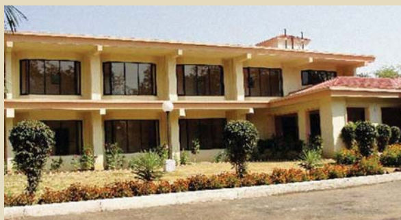
New Satpura Rest House
