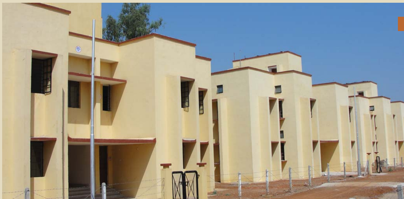
Newly built Type-II quarters
